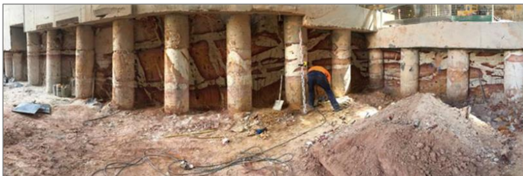
Figure 5: View from the first stage of excavation for a basement within the GPO Fault Zone ([6]).
